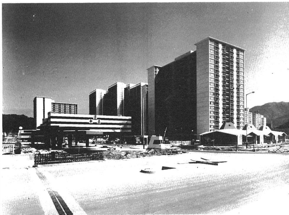
Mei Lam Estate—Phase 1, Sha-Tin New Town (General View)
