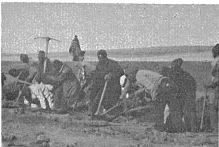
Pick and shovel excavation is proving very effective in Lesotho
